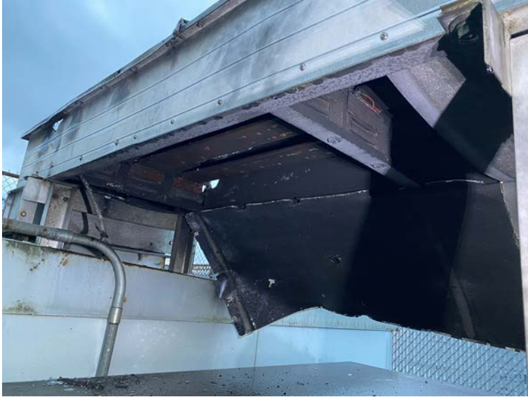
Original Central Substation Failure - November 2020
